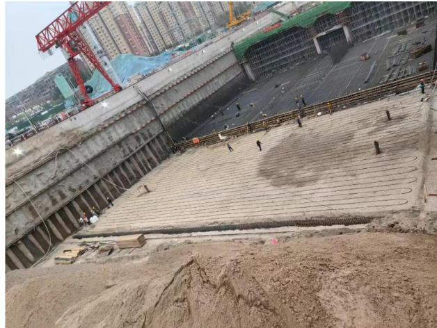
Figure 3. Construction Site of the Snow-Melting and De-Icing Section in the Energy Tunnel [39]
